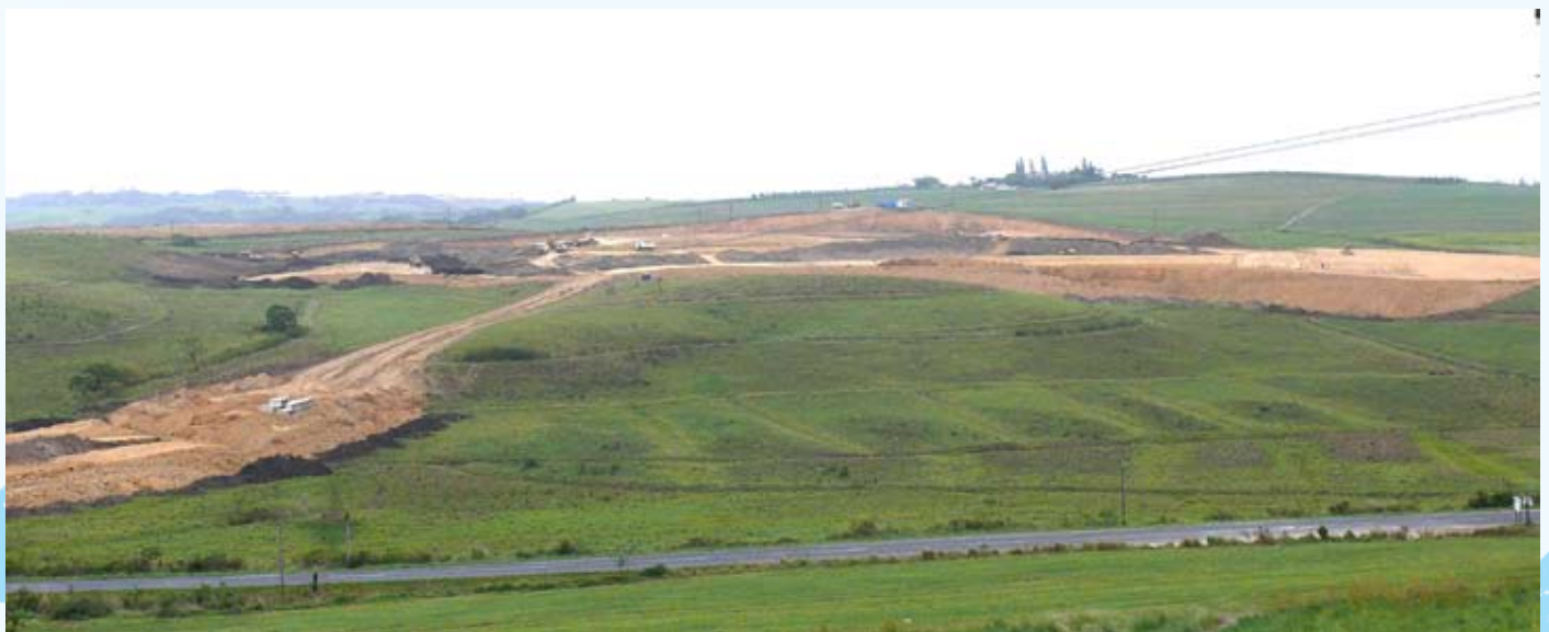
Ugu Sports and Leisure Centre site
